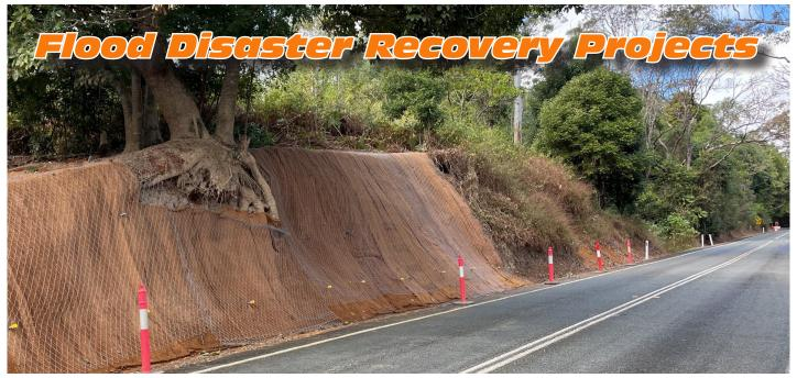
Reconstruction works are occurring across multiple Gold Coast and Scenic Rim roads following heavy rainfall in December 2020 and March 2021. Reconstruction works include road rehabilitation and slope stabilisation. Assistance will be provided through the jointly funded Commonwealth-State Disaster Recovery Funding Arrangements (DRFA).
