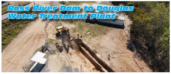
**Townsville City Council** has engaged **CivilPlus Constructions** to construct a 9.5km pipeline from Ross River Dam to the Douglas Water Treatment Plant. The purpose of this project is to duplicate the existing aging pipeline and enhance Townsville's water security. When complete this new pipeline is expected to provide 85% of the city's water supply.
